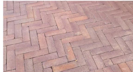
Example of new brick paving
